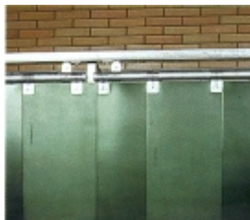
Rocker clips facilitate opening and closing. Wear and tear due to bending stress is avoided.
